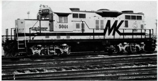
Morrison-Knudsen Railroad Equipment Leasing Co. 5001 (see August Newsletter) is seen at CP Rail's St. Luc Yard, Montreal, July 5, 1980. The locomotive, a former UP GP9 with a Sulzer prime mover, was tested by CP Rail from July 5 to July 15.
