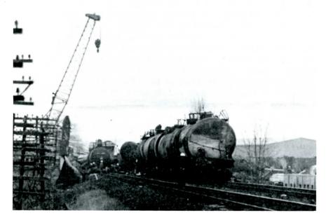
Damaged cars on the eastbound track, while the westbound track is used as access to the wreck site. The crane, left, is the Nadrofsky Steel Erecting crane often used in serious derailment cleanups. Beyond is a CP auxiliary working from the east end.
