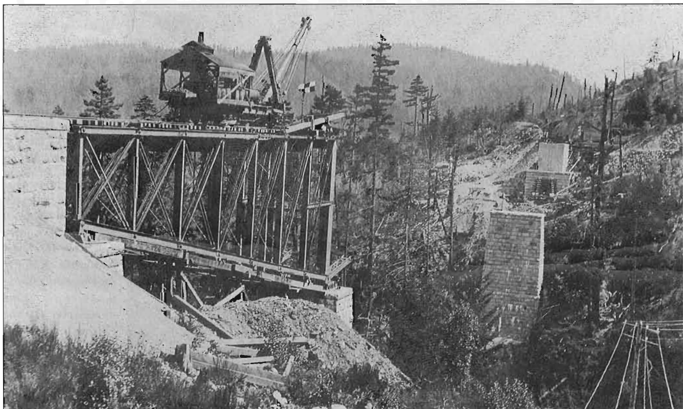
The Cisco Bridge has been dismantled and moved to the Esquimalt and Nanaimo Railway where it is being reassembled (and lengthened) over the Niagara canyon. CPR Archives # a26246
