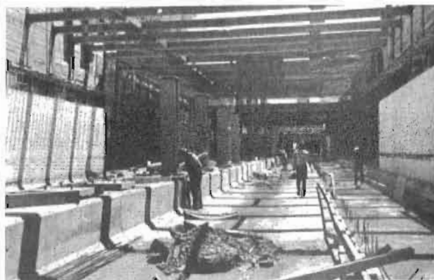
ABOVE: Concrete work progressing steadily in the area of Wellesley Station. Note the steel reinforcing bars ready to be placed in the concrete.
