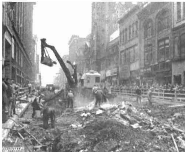
Excavation on Yonge Street, looking north from Queen. In the foreground air hammers are breaking up the soil.
