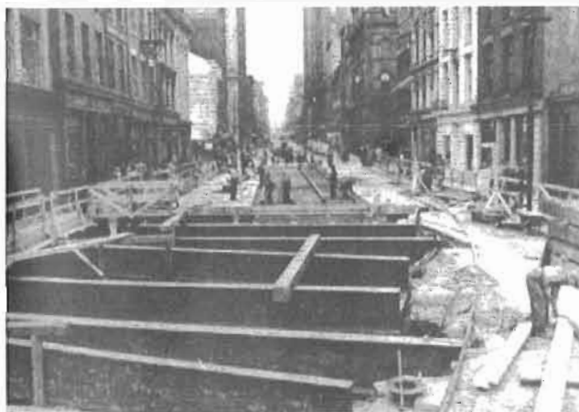
This photo illustrates the "cover" part of "cut and cover". It is taken on Yonge Street, looking north to Wellington, and shows the steel deck beams in place in the foreground, with timbering and laying of temporary street car tracks in the background.
