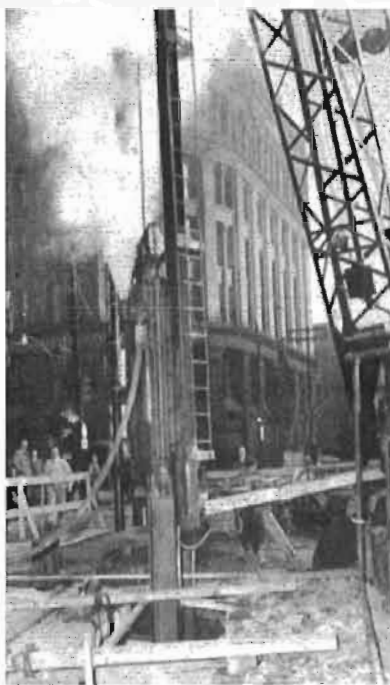
A pile driver in action on Front Street looking east, in the early stages of the work.
