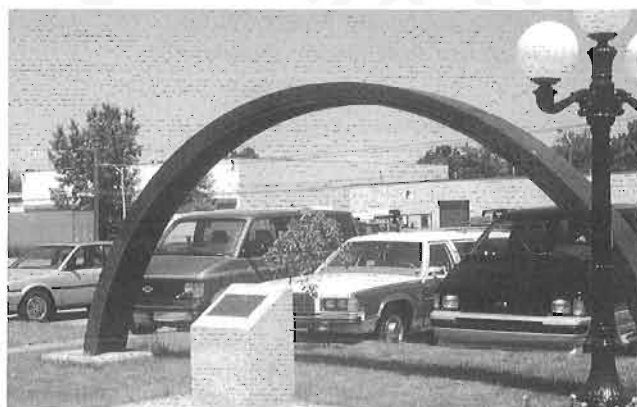
The monument at Sarnia to commemorate the St. Clair tunnel, seen on June 12, 1991. It is made from actual spare sections of the tunnel lining, kept in storage for 100 years.
