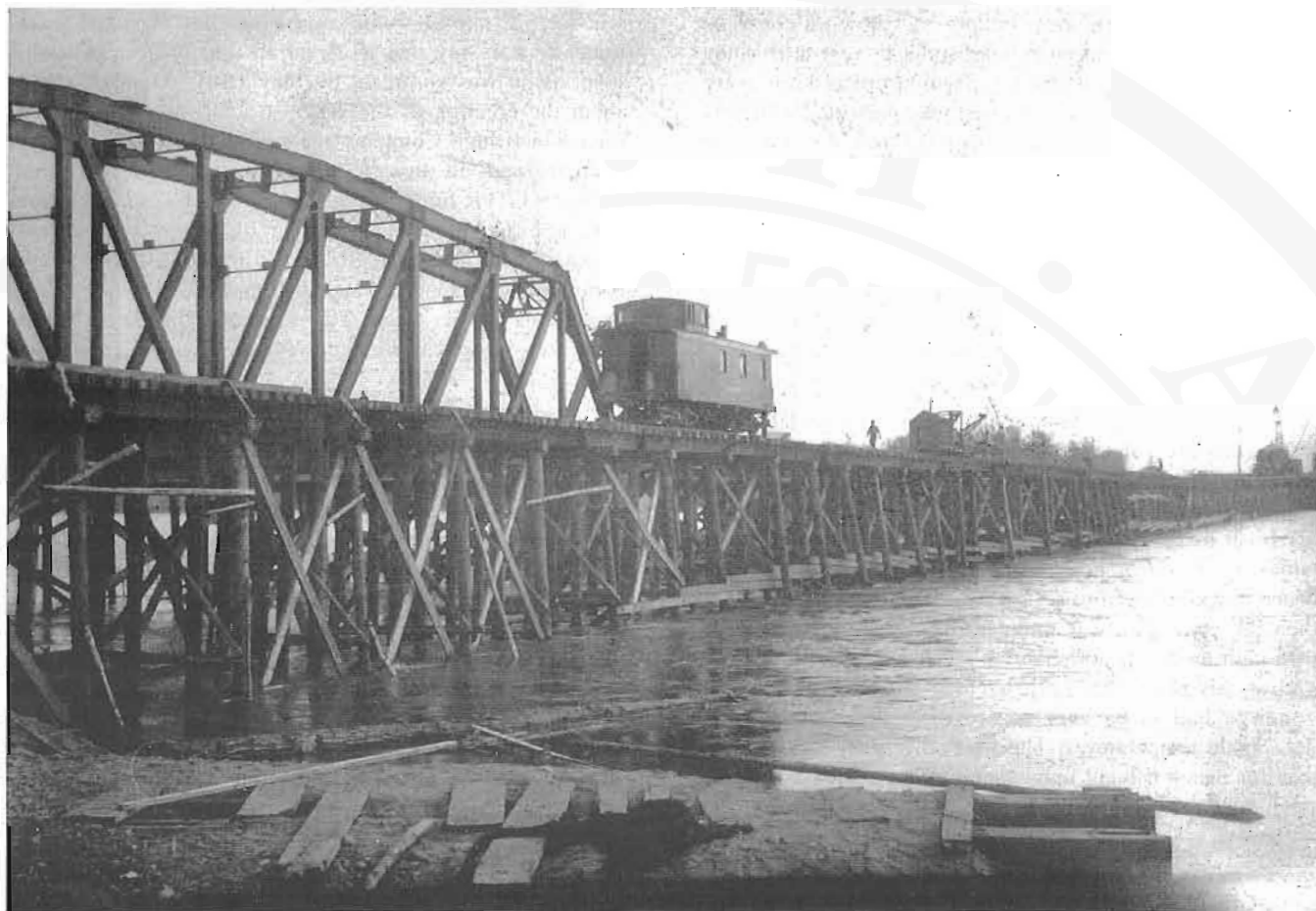
View taken from the west bank of the Fraser River looking upstream on a date presumed to be in mid-1914. Span No. 13 has been erected. The river is in flood.
