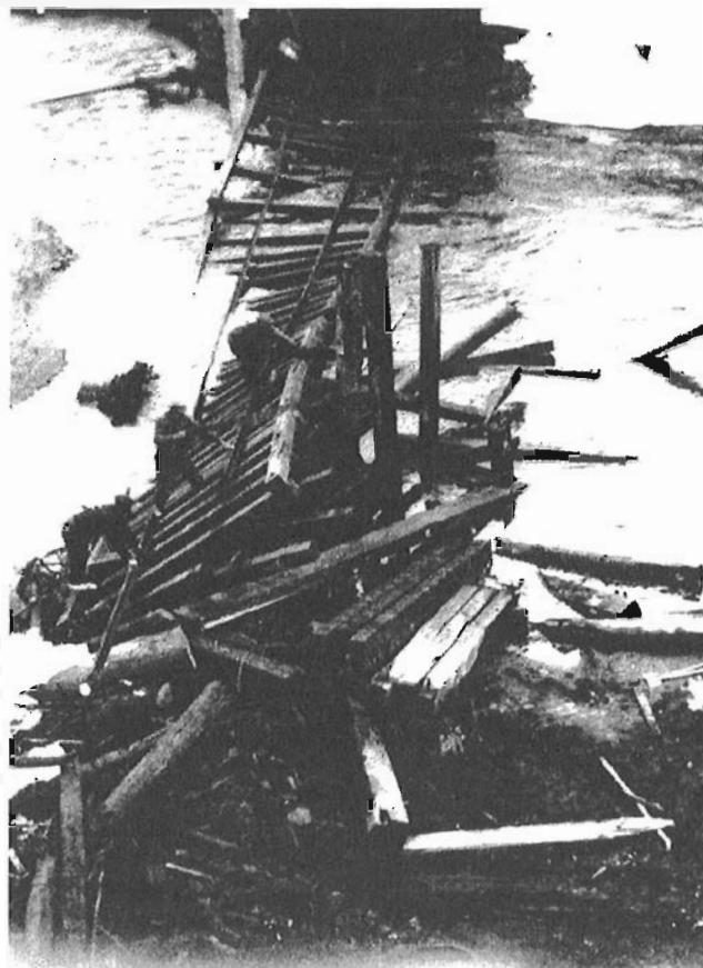
No. 72787 - CNER, the old sections of the original bridge over the Bear River were sawn up & pulled down to allow reconstruction of a new bridge to replace it. Note the men climbing on the twisted rails over the rushing river
