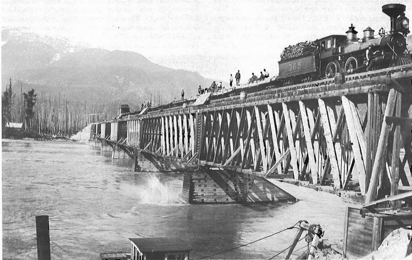
The second CPR bridge inspired much greater confidence concerning its capacity to handle heavily loaded trains. Locomotive #365 heads up the work train dropping rock at the base of the piers. Locomotive 365 was built in July 1886 by the Canadian Locomotive Company at Kingston, Ontario. Its career lasted more than 40 years as it was not taken off the roster until October 1926.
