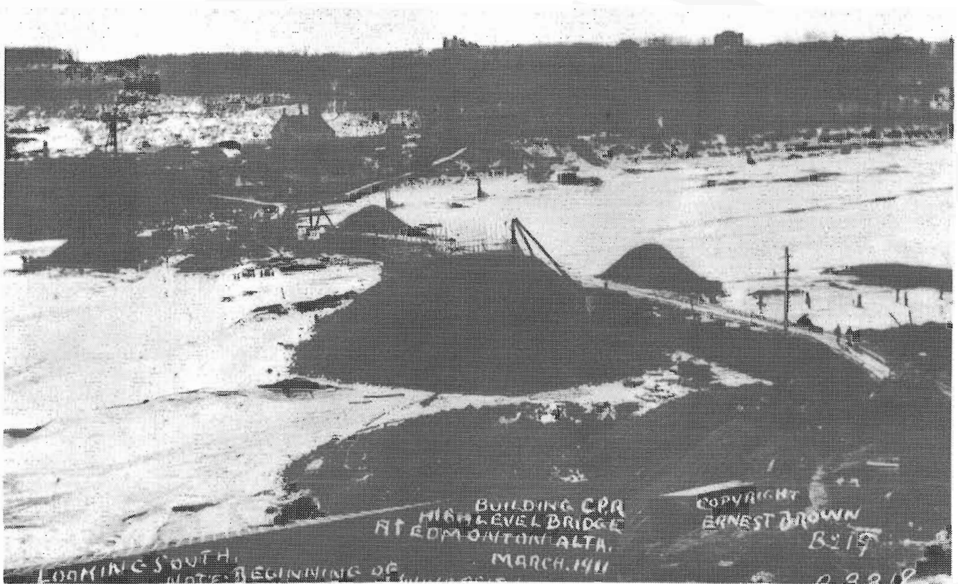
The pier excavations are well under way in this view looking south in March 1911. Almost ready for the frameworks for the concrete pouring.
