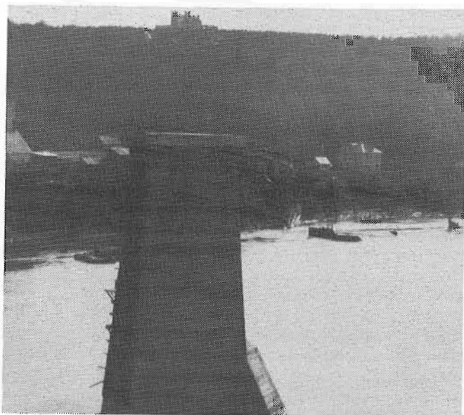
One of the 125-foot piers all ready for the steel. In the background is St. Stephen's college, one of the first of the University of Alberta buildings.
