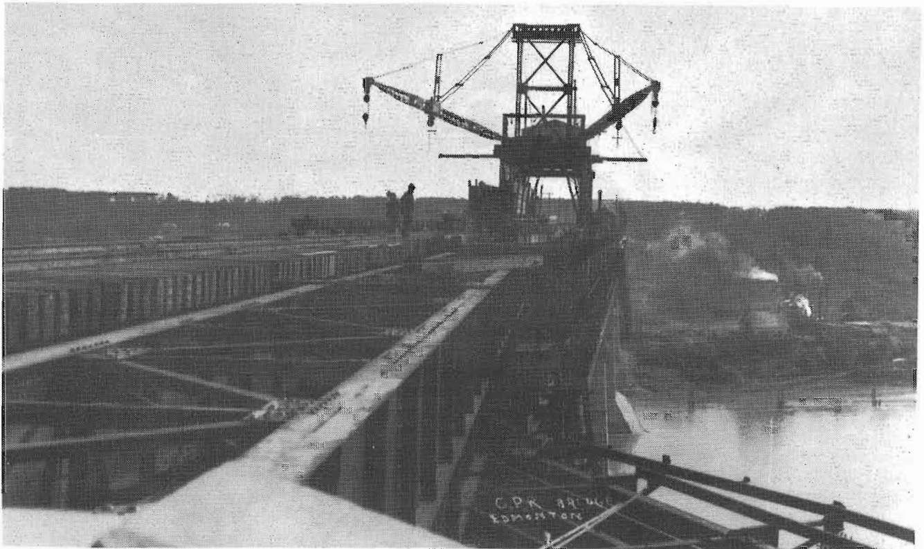
This is a good view showing the traveller used in the construction. It was arranged to erect not only the main spans but also the other spans without falsework. The rigid arms are extended to counterbalance the high winds in the valley. The sidewalk and roadway are below.
