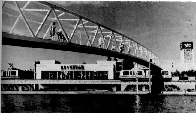
Artist's concept of the GO URBAN station at Ontario Place on the CNE test installation. Stations will be "off-line" to permit cars or trains to bypass the station when a stop is not called for.
