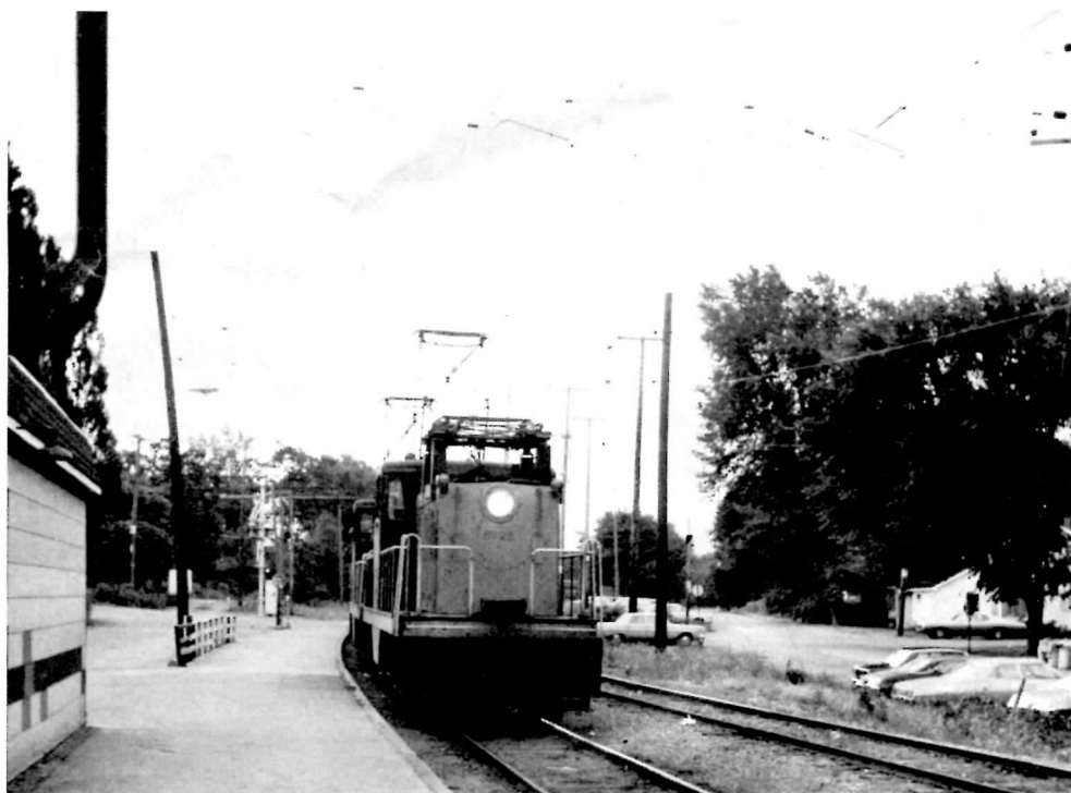
ABOVE:Val Royal is the junction of the Mt Royal and the Montford Sub- divisions.6749 trails train 961 for Deux Montagnes,the end of the line. RIGHT:6725,27,class Z-5-a leading train 951 into Deux Montagnes.The engines were two of three built by General Electric in 1950.Ordered as 9200-02,they were delivered as 200-02 and later renumbered 6725-27. (Both R. Lampkin)
