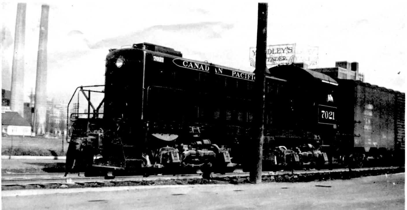
A study in early Canadian Pacific Diesel Yard Power. All are Alco model S2 and wear the first CP switcher paint scheme of tuscan red, black lozenge with gold lettering and trim. All were taken along the Toronto waterfront in the late forties and are part of the J.T.A. Smith/U.C.R.S. Collection. Featured here are CP 7029 (DS10c ALCO 1945), CP 7026 (DS10c ALCO 1945), CP 7021 (DS10b ALCO 1944), CP 7014 (DS10a ALCO 1943) CP 7022 (DS10b ALCO 1944).
