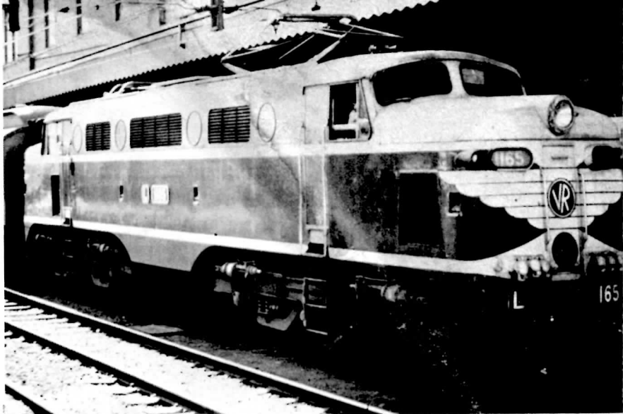
RIGHT: Double end electric locomotive L1165 shot at Flinders Street Station Melbourne Australia, 25 Dec. 73. The engine is one of a series used by the Victorian Government Railways (VR) and is 5'3" gauge, 1500 VDC (ICP). BELOW: Amtrak Metroliner 807, still in Penn Central colours with an Amtrak painted Metroliner behind it, approaching Philadelphia's 30th Street Station. (RWL)
