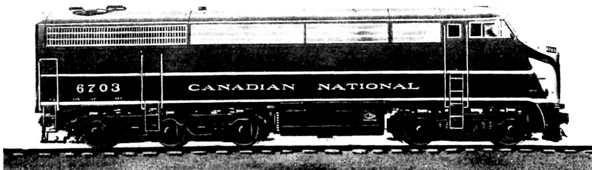
This Diesel-Electric Passenger locomotive (A unit) (Class CPA-16 — Road Numbers 6700-6705) was built for Canadian National Railways by the Canadian Locomotive Company in 1955.
