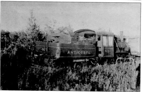
No. 2, was a Heisler, except it was new and had 36" drivers and 13 x 12" cylinders. No. 3 was out of service between 1923 and 1926. It was reported to have been back in service between 1926 and 1934, and was scrapped as part of the 1939 scrapping.
