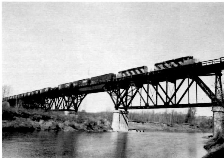
CN SD40s 5127 and 5112 crossing the Pembina River immediately west of Sangudo, Alberta, on May 6, 1994, eastbound from Whitecourt to Calder Yard in Edmonton. The trestle, truss, and girder spans make an interesting combination.
