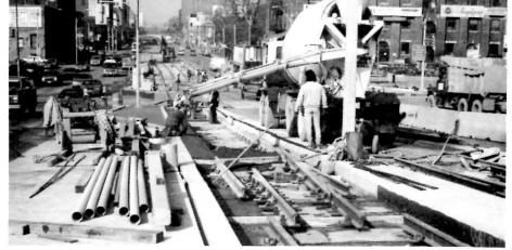
Construction crews took advantage of one of the breaks in winter in late January, 1990 to complete track laying on Spadina Ave. for the Harbourfront LRT connection to King St. In this scene, looking north to Front St., note the special rail with expansion joint about to be installed, the centre pole for the overhead, and the unloading platform, left. Only a small amount of concrete pouring remained to be completed here by late February.
