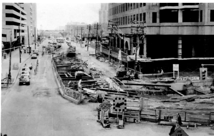
TTC Harbourfront LRT construction, looking west along Queens Quay at Bay St., from the walkway between the Harbour Castle Hotel and Convention Centre. At this point the line leaves Queens Quay Station (beneath Bay, right), turns west, and climbs a ramp to the surface. Construction in this area should be finished near the end of summer.
