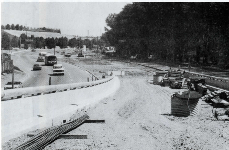
Construction progress on Calgary's Northeast LRT Line: this view looking outbound shows the ramp leading down from the new Bow River Bridge, and the median strip in the middle of Memorial Dr. in which the tracks will be laid. July 10, 1983. The line is scheduled for opening in 1985.
