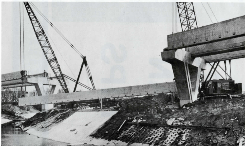
One of the beams which will carry the TTC Scarborough RT line is lowered into place at the point where the line follows Highland Creek briefly, east of Midland Ave. Photo taken March, 1983. View looks south.
