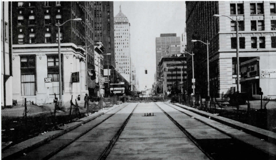
This view shows the new LRRT tracks of the NFTA on Main St. in downtown Buffalo, looking north at Swan St. The photo was taken in October, 1982, shortly after the rails had been laid, then embedded in poured concrete. This spring the poles for supporting the overhead will be installed in the space between the tracks.
