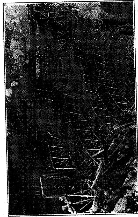
Fig. 4. The steel truss completed, with the greater part of the timber of the original structure still in place.
